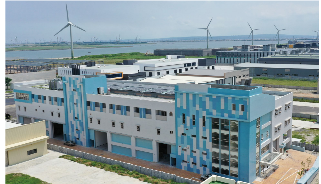
TCC Group's Self-Built Renewable Energy O&M Center
