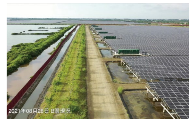
Completing the greening of the embankment
