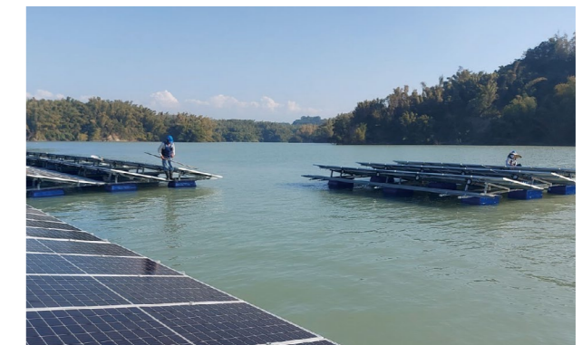
Modules are being moved to their positions
